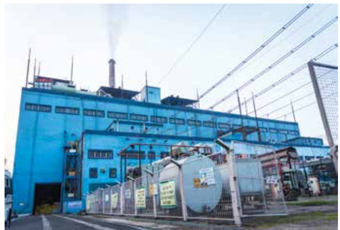
Service Building NSPCL Durgapur
