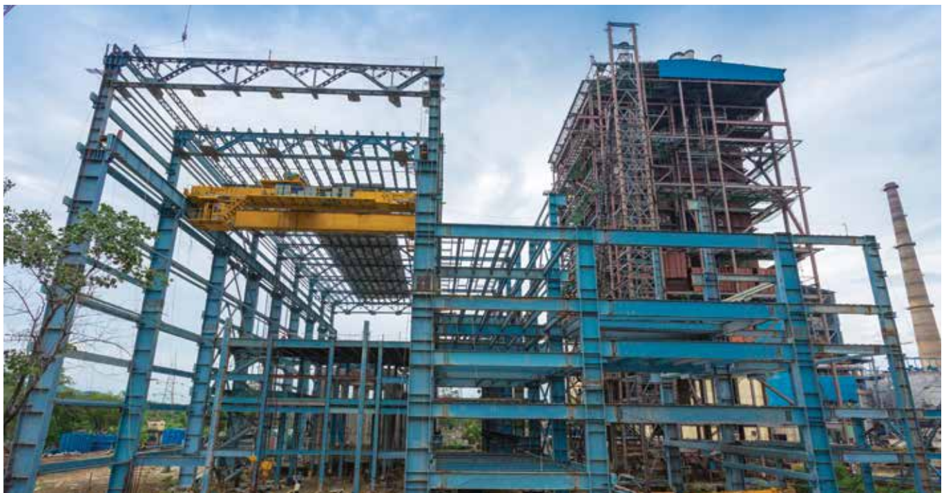
New Project Construction - Rourkela
