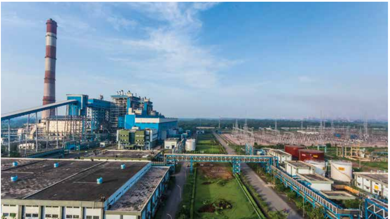
Panaromic View Bhilai Expansion Project
