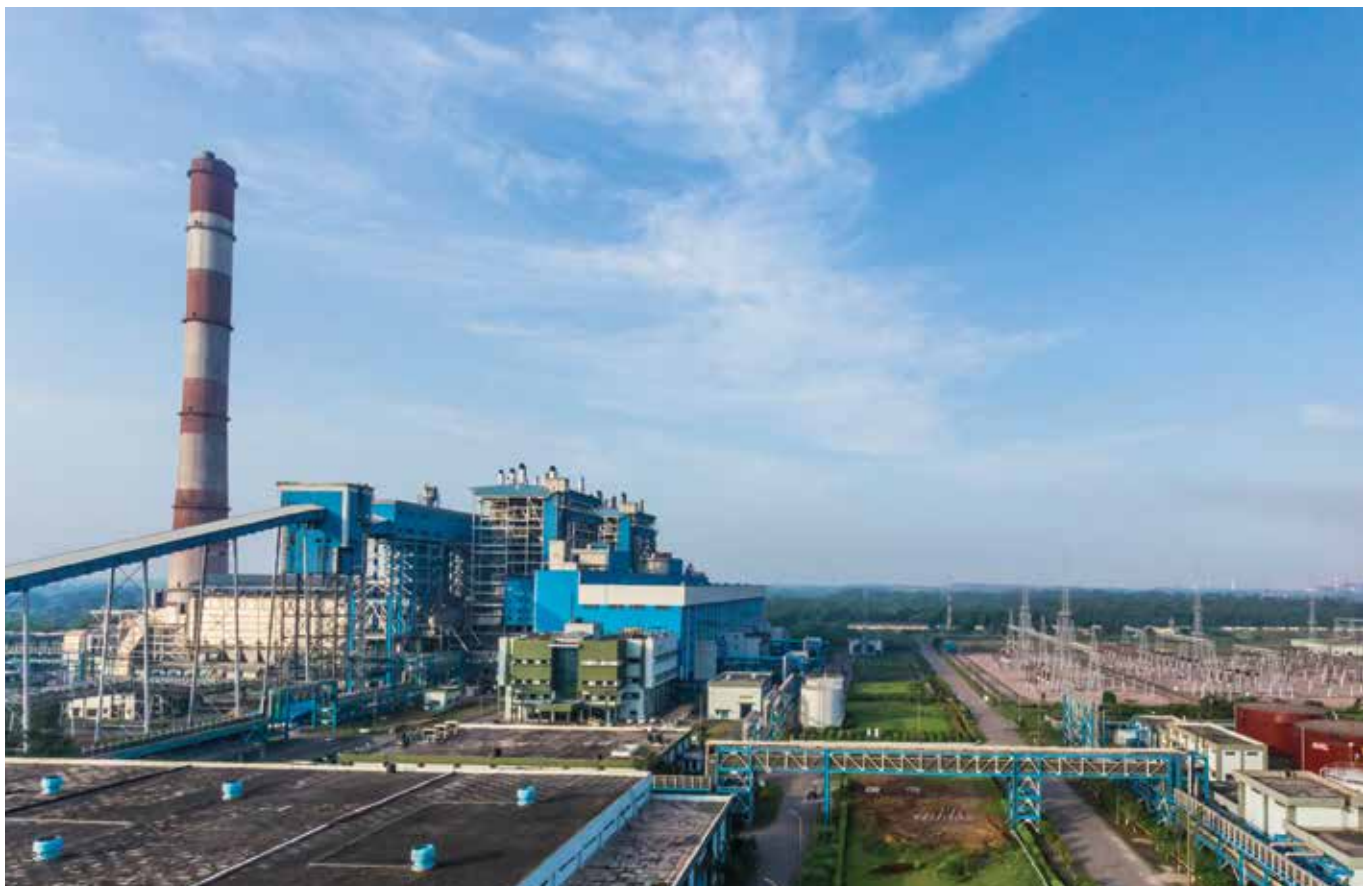
Panoramic View Bhilai Expansion Project
